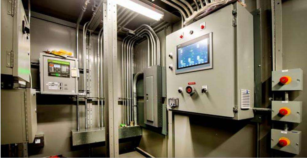
Onboard paralleling between three MTU Onsite Energy 16V 2000 DS generator sets ensure emergency power supply for Gracedale's 365-acre nursing home facility.
