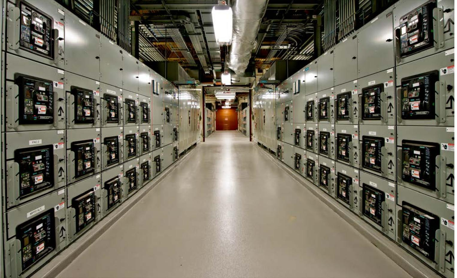
A sophisticated control system of Siemens PLCs coordinates the seamless operation of seven generator sets, four switchboards and two utility sources.
